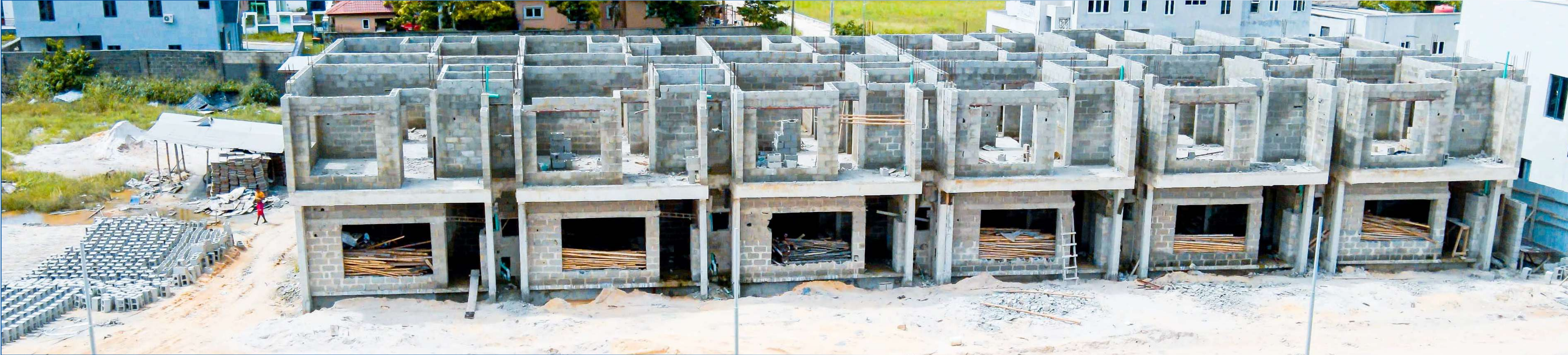
Ongoing Construction of the terraces
