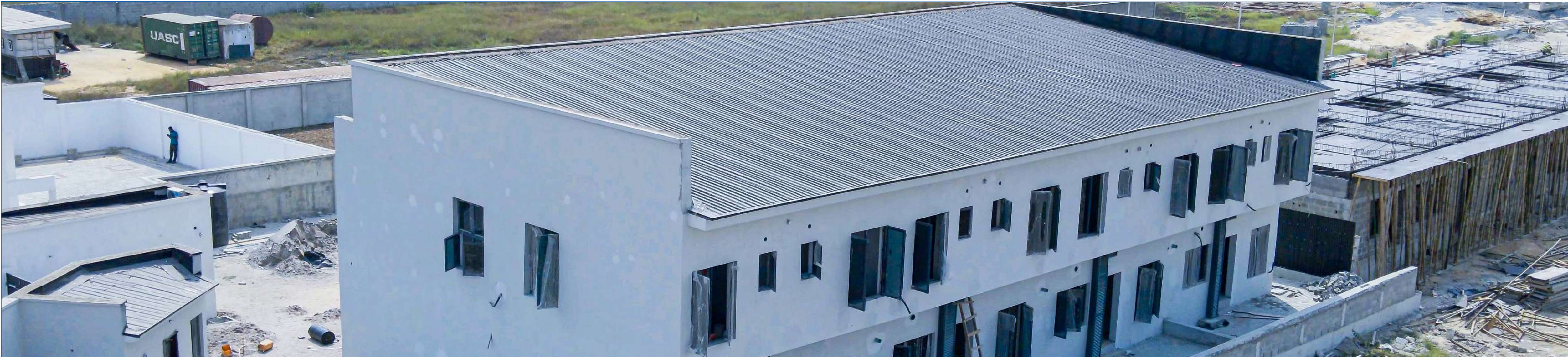
Rear view of Terrace construction
