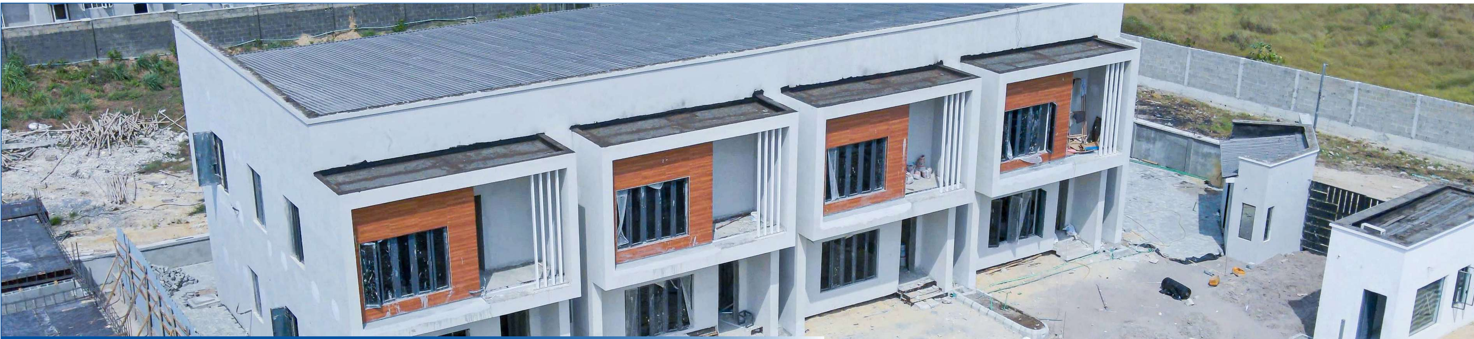
Front view of Terrace construction
